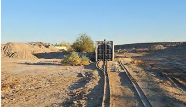
And here is a drive-in engine house (Left)
